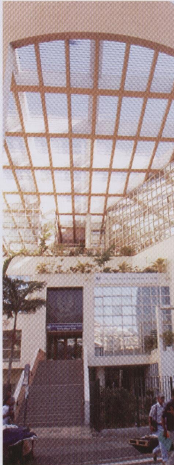
CSO in the LIC Building
